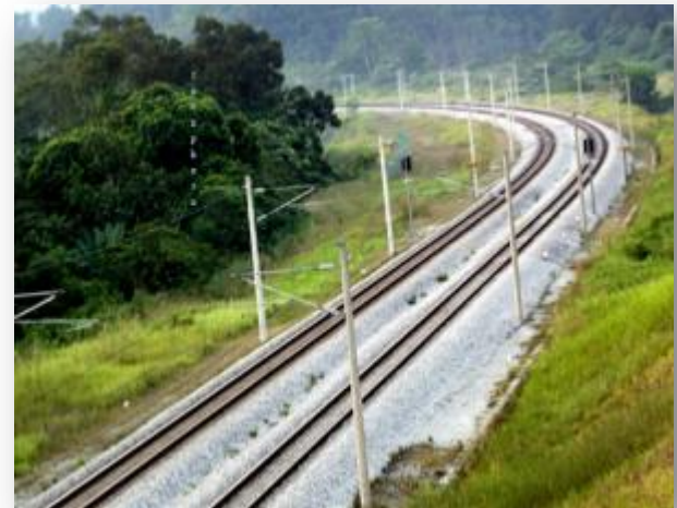
Double Track Railway
